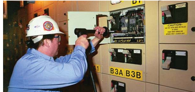
MCCB testing using the HCP2000
