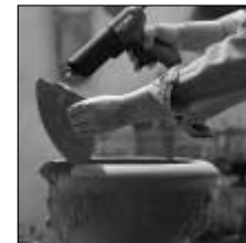
e.g. repairing planter
