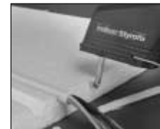
Cutting U-sections in insulation boards for embedding cables
