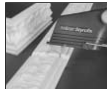
Neatly cutting lengths of coving
